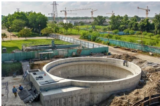
GRAVITY THICKENER TANK
