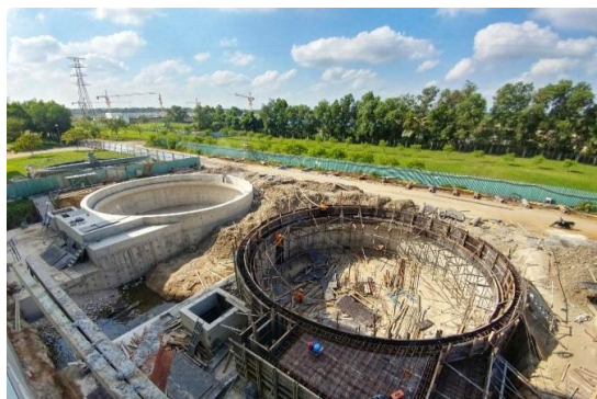
GRAVITY THICKENER TANK
